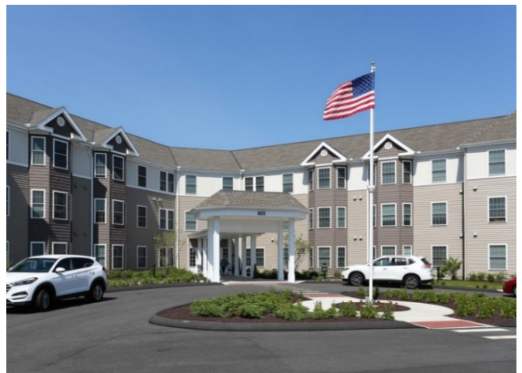
Victoria Gardens in Waterford, CT, which contains mixed-income housing, was constructed with assistance from LIHTCs. Photo: Affordable Housing Online
